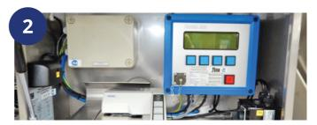
FLOWCOM 2000: flow metering system operating on the basis of effective pressure measurement, most often used in Germany and Austria.
