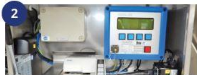
2 FLOWCOM 2000: flow metering system operating on the basis of effective pressure measurement, most often used in Germany and Austria.
